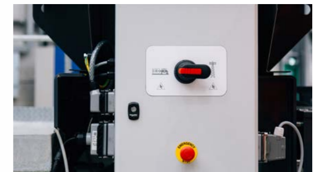
Change over switch as standard to allow the use of onsite mains power
